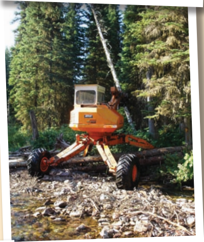
A helicopter and spider excavator were used to build large wood structures designed to provide bull trout habitat, trap spawning gravels, and increase channel complexity
