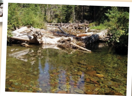
An example large wood habitat structure following construction (above) and three years after construction (right). This structure accumulated more wood and generated channel scour, providing cover for juvenile bull trout and other species.
