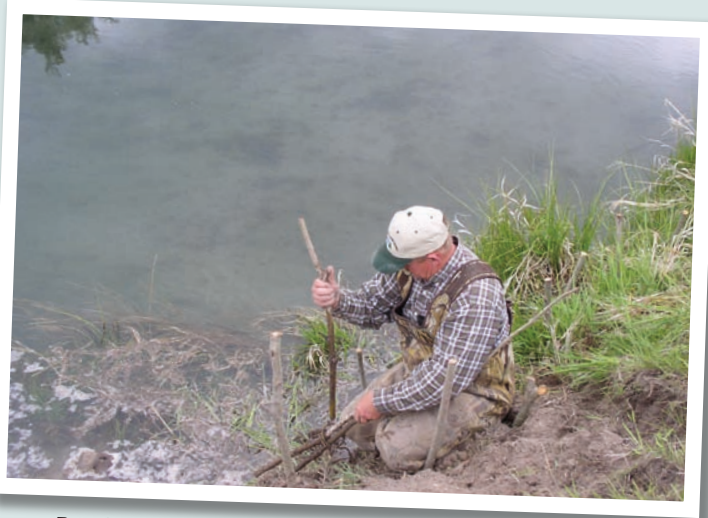
Pete Woll installs willow stakes on Mill Creek Restoration site
