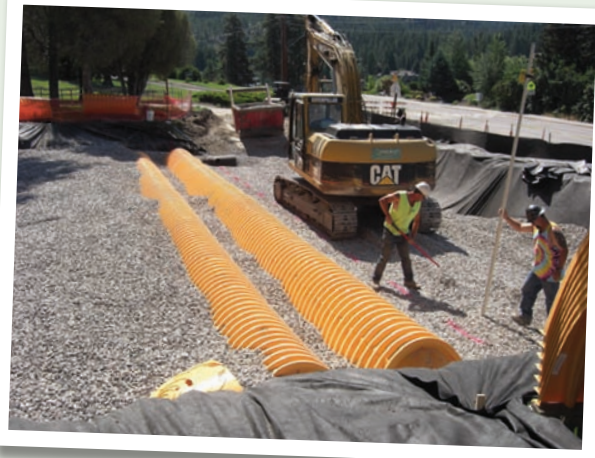
Stormtech detention/filtration system during construction at Bigfork School District
